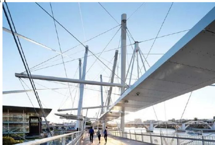
Fig. 1: Kurilpa Bridge, Brisbane (Australia), is the world largest tensegrity bridge
